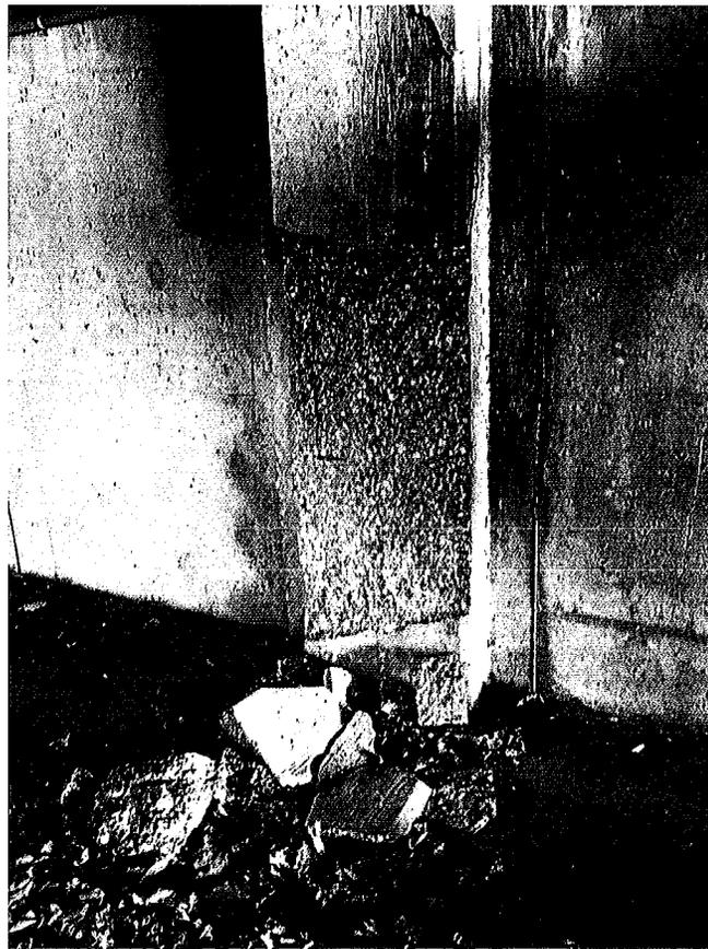
Photo 1. Concrete pier spall on grids WC/W11
