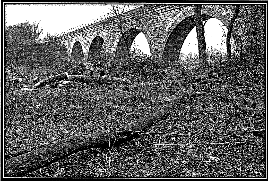
5 Arch Bridge Work day 3-15-2017
