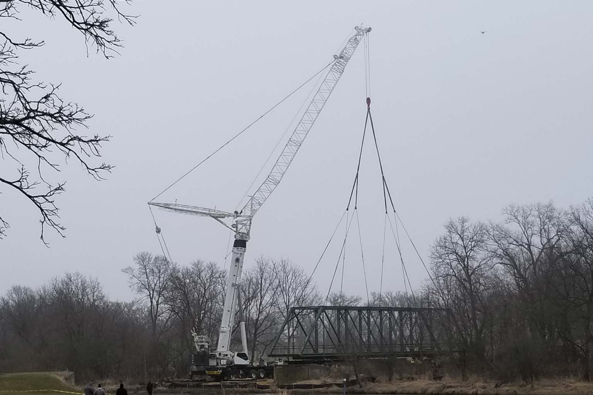
S. Smith Road Bridge - (Fed. Aid)
