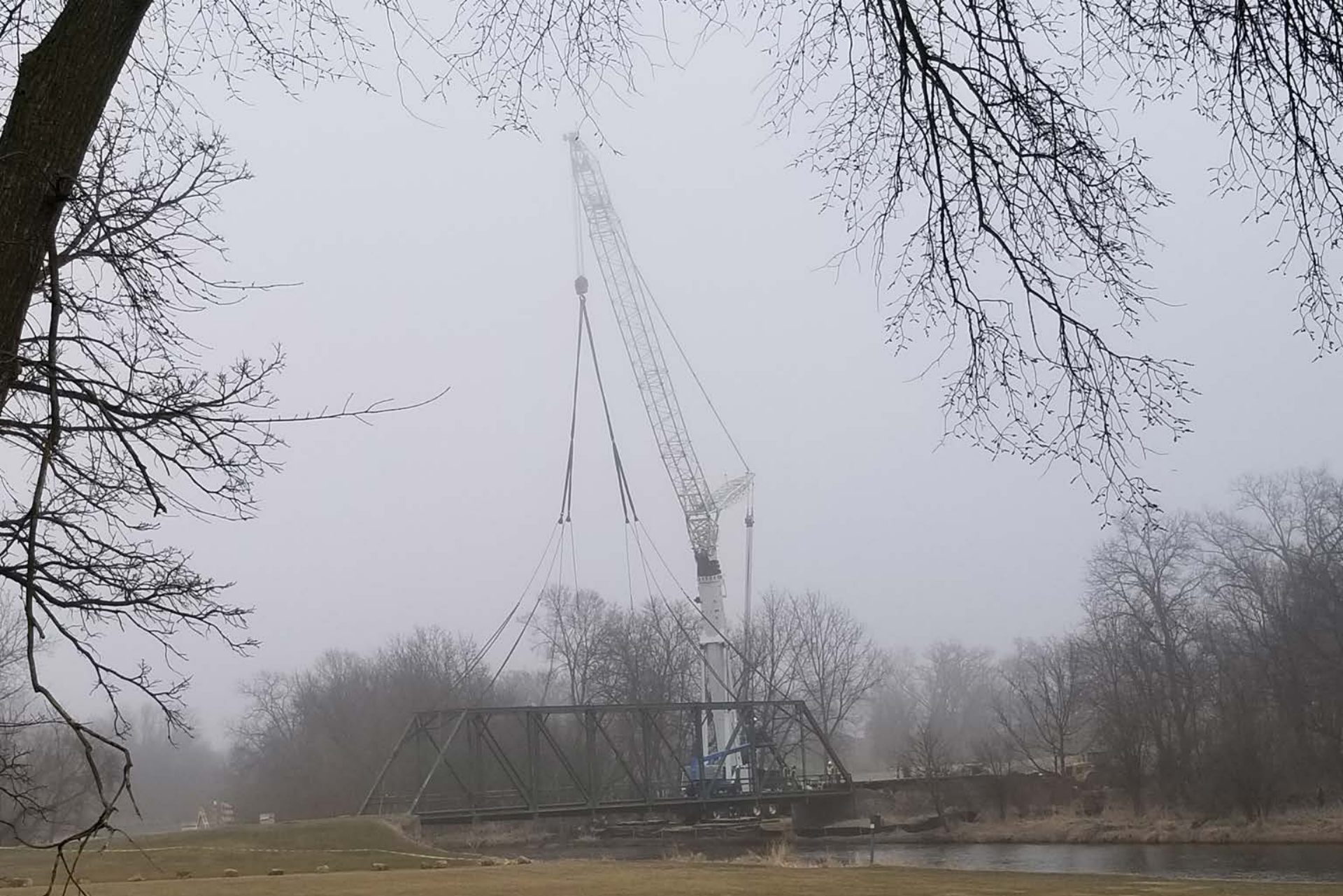
S. Smith Road Bridge - (Fed. Aid)
