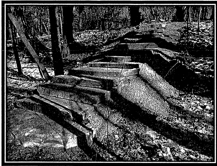
Carver Roehl Erosion Control Project
