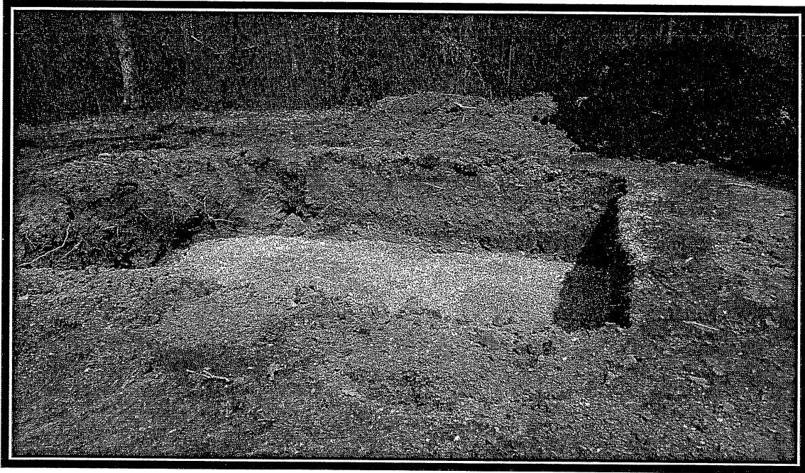
New Bathroom Install at Carver-Roehl
