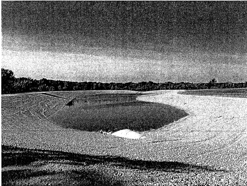
Photo 1: Completed pond and northern concrete pipe outlet (Looking South) (06/19/15)
