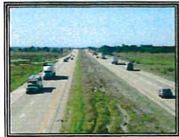
State Trunk Highway System
