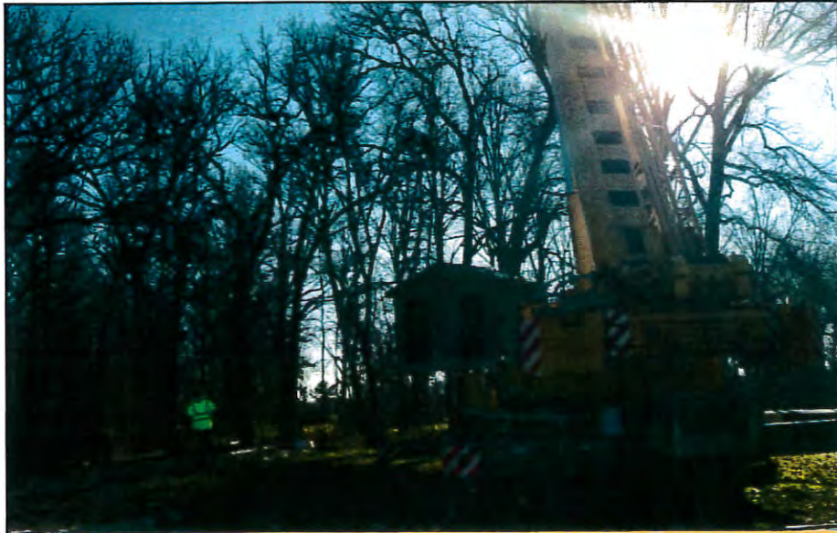
Happy Hollow Restroom Install
