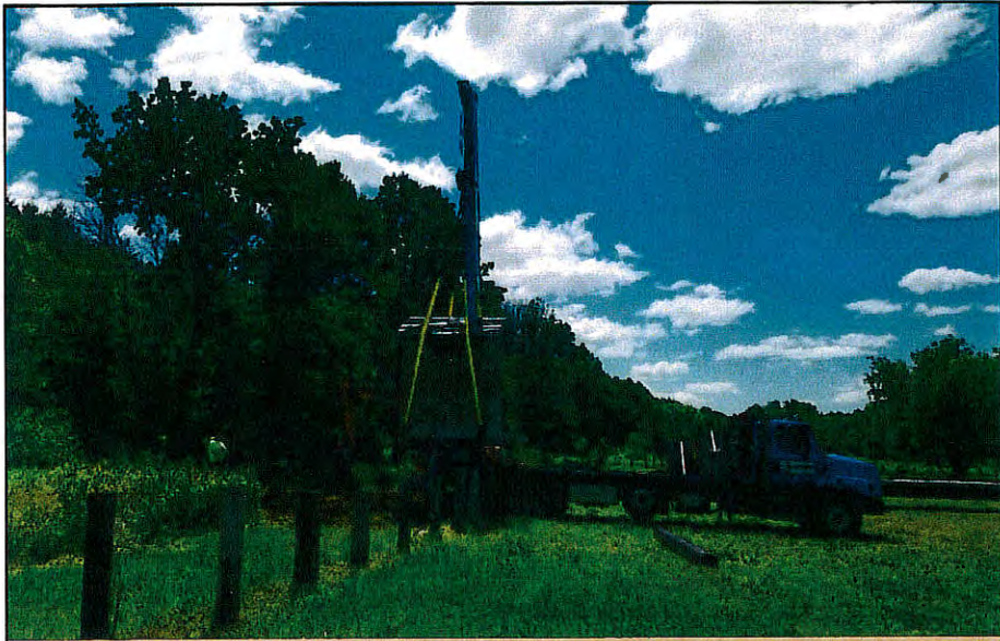
Gibbs Lake Restroom Install
