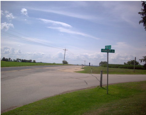
Facing south on CTH F at Pomeroy Road. Inadequate site distance.
