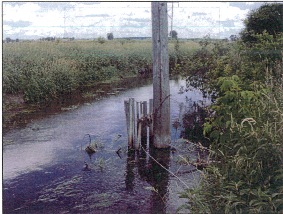
Photo 4. Photo viewing downstream at pole structure exposed within Bass Creek (June 2011).
